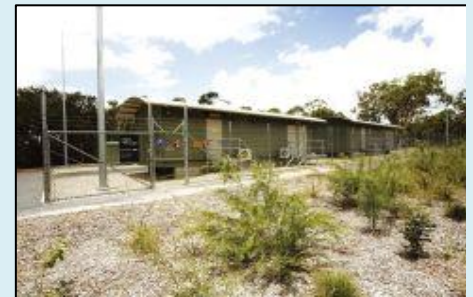
Figure 1: Above is an example of a Zone Substation. Development within 100 metres of this site would trigger referral to us.
