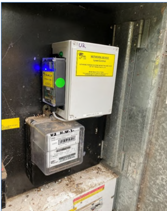
Load control relay and comms device in-situ
