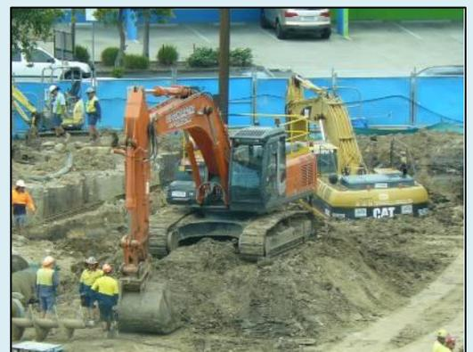
Filling works over underground cables can reduce the operating capacity and increase faults. This can also impact other assets within the network and subsequently incur additional maintenance and upgrade costs. Prior to the works starting, a cable rating assessment must be done to identify the operating limits of underground assets and ensures the network capital expenditure is spent appropriately.
