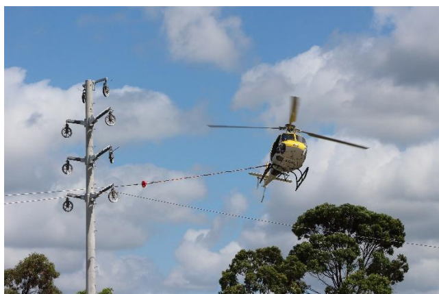
A specialist helicopter and highly skilled crews will be stringing wires for the new major powerline from the air.
