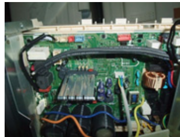
After removing the connectors
