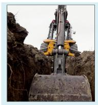
Excavation works close to substation boundaries can cause earth movement around compound foundations, compromise protective earth grids and cause high voltage cable damage or exposure. These can all impact on the performance and safe operation of a substation and can be time consuming and costly to rectify.
