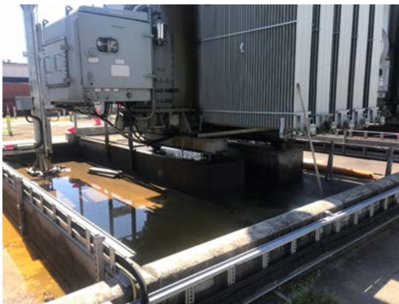
Figure 9: Transformer TR2 showing leaks and water with oil in the bund
