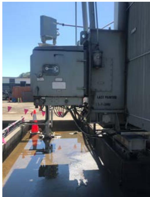
Figure 11: Transformer TR3 showing leaks and water with oil in the bund
