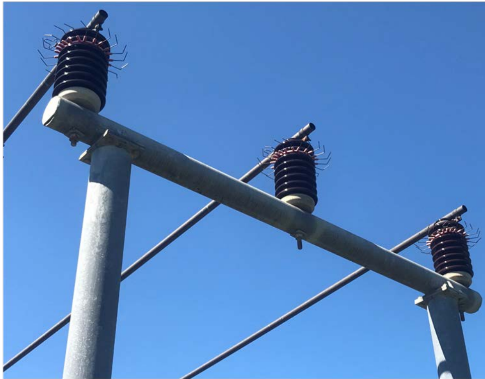
Figure 14: Ageing 33kV bus support insulators
