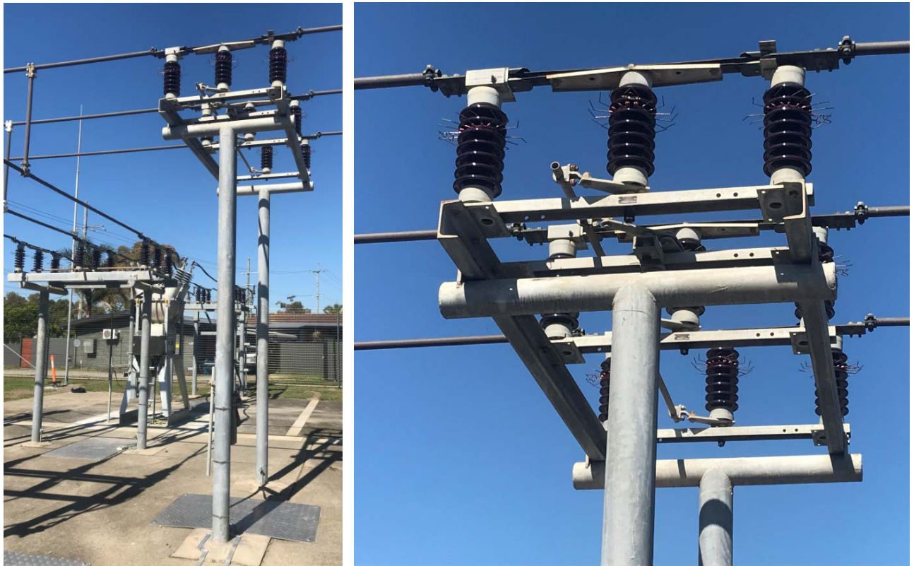
Figure 16: Views of 33kV horizontal double-break type isolators
