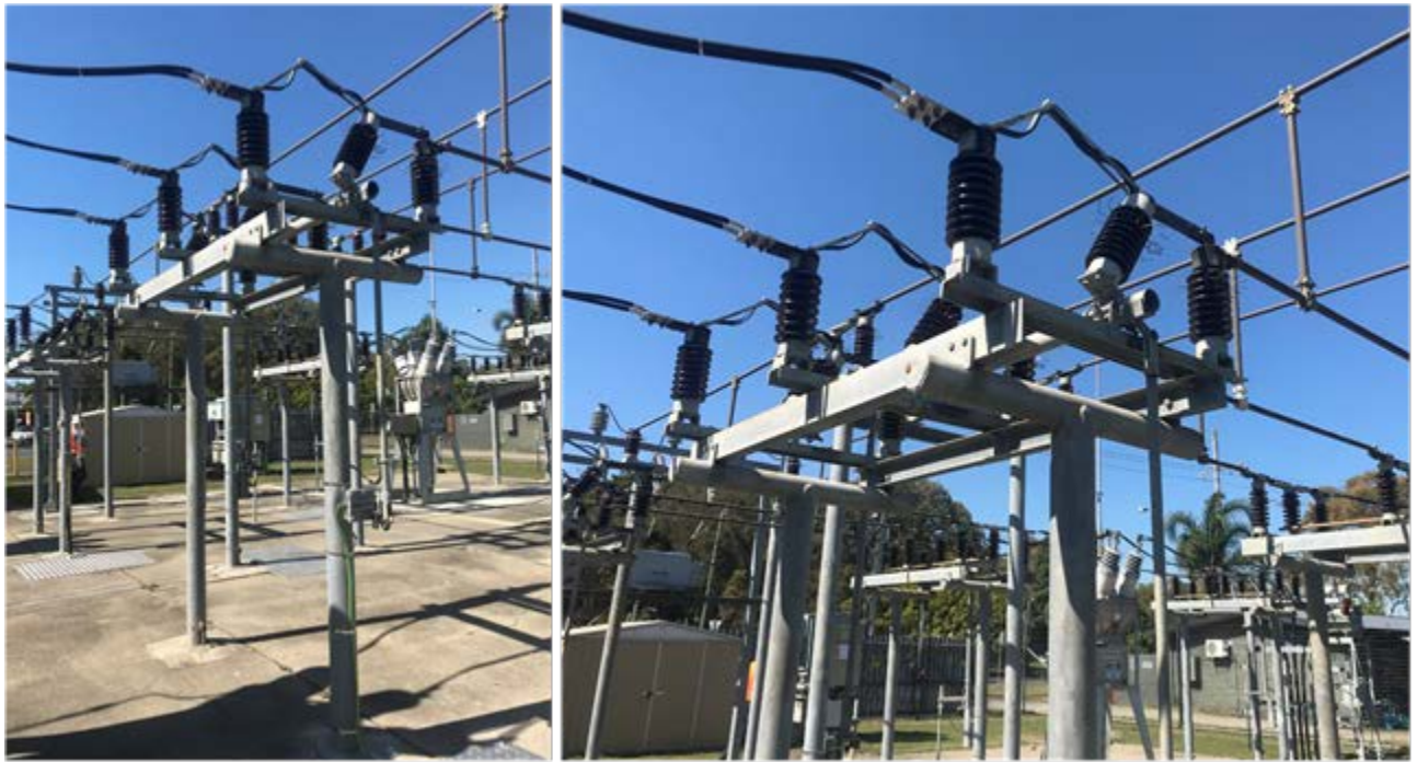
Figure 13: Views of 33kV braid type isolators
