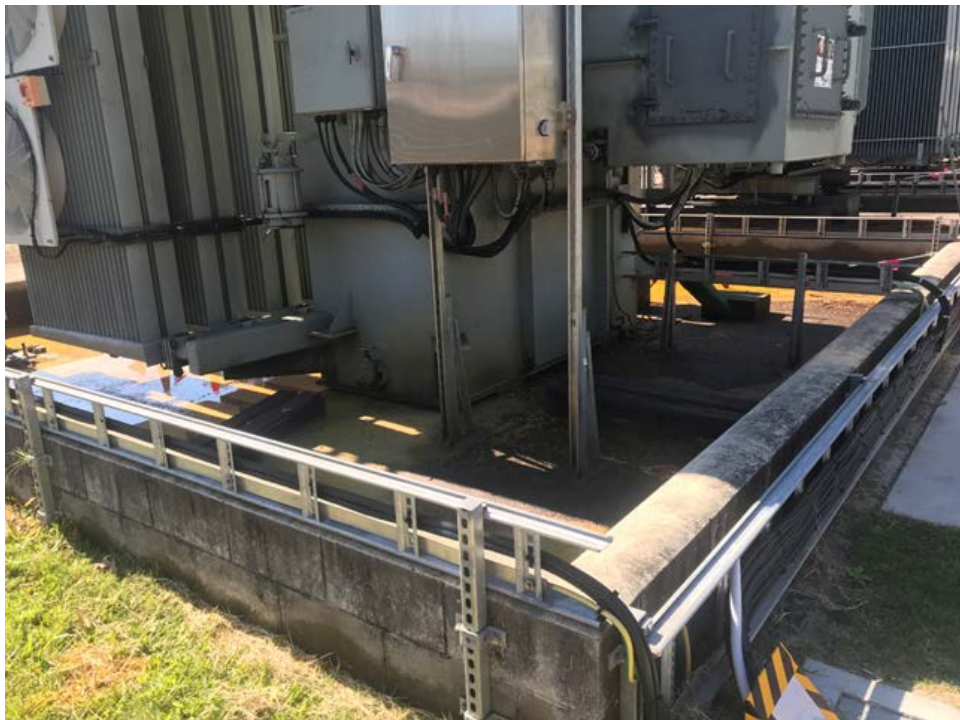
Figure 7: Transformer TR1 showing leaks and water with oil in the bund
