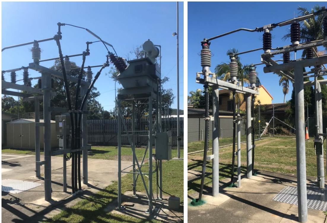
Figure 15: 33kV feeder cable terminations (396 on left and 3756 on right)
