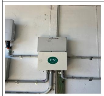
Correct installation in alternative enclosures where panel space is limited.
