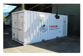
The CESS Stage 1 project was completed in 2017 and involved the development of a centralised inverter and energy storage test platform (83kVA/200kWh). The CESS Stage 2 is an application of the CESS platform using advanced control systems. The project investigated applications for the distribution network and isolated systems, considering the challenges and benefits of DER solution to power quality, capacity and renewable enablement.
